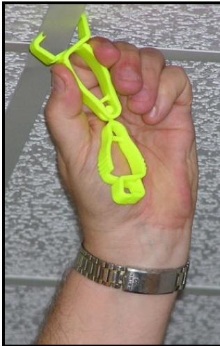
Squeeze and attach large end of Handi-Klip® to main line of ceiling T-grid.
